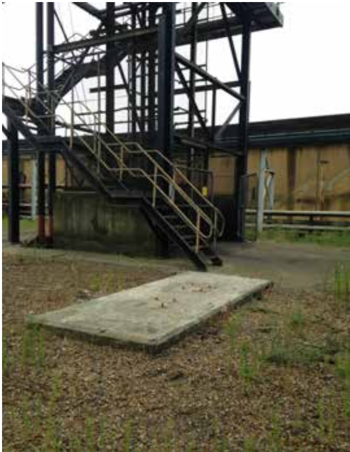
Plate 5: West facing photograph of rectilinear building in the eastern boundary of the study site with steps accessing the conveyor belt in the foreground
