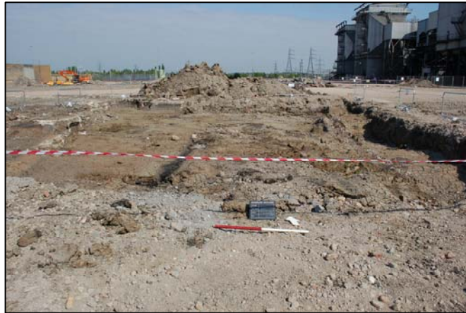
Area 2C, looking north
