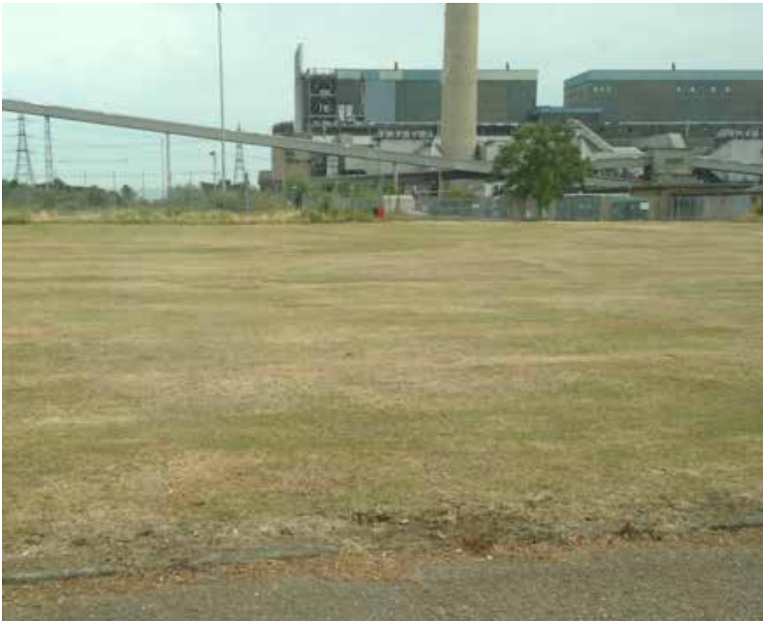
Plate 24: East facing photograph of levelled former sports pitch to the north of Tilbury A
