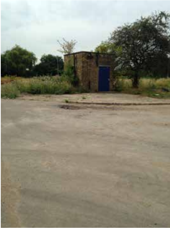
Plate 3: Small single storey sub-station in the south-east of the site
