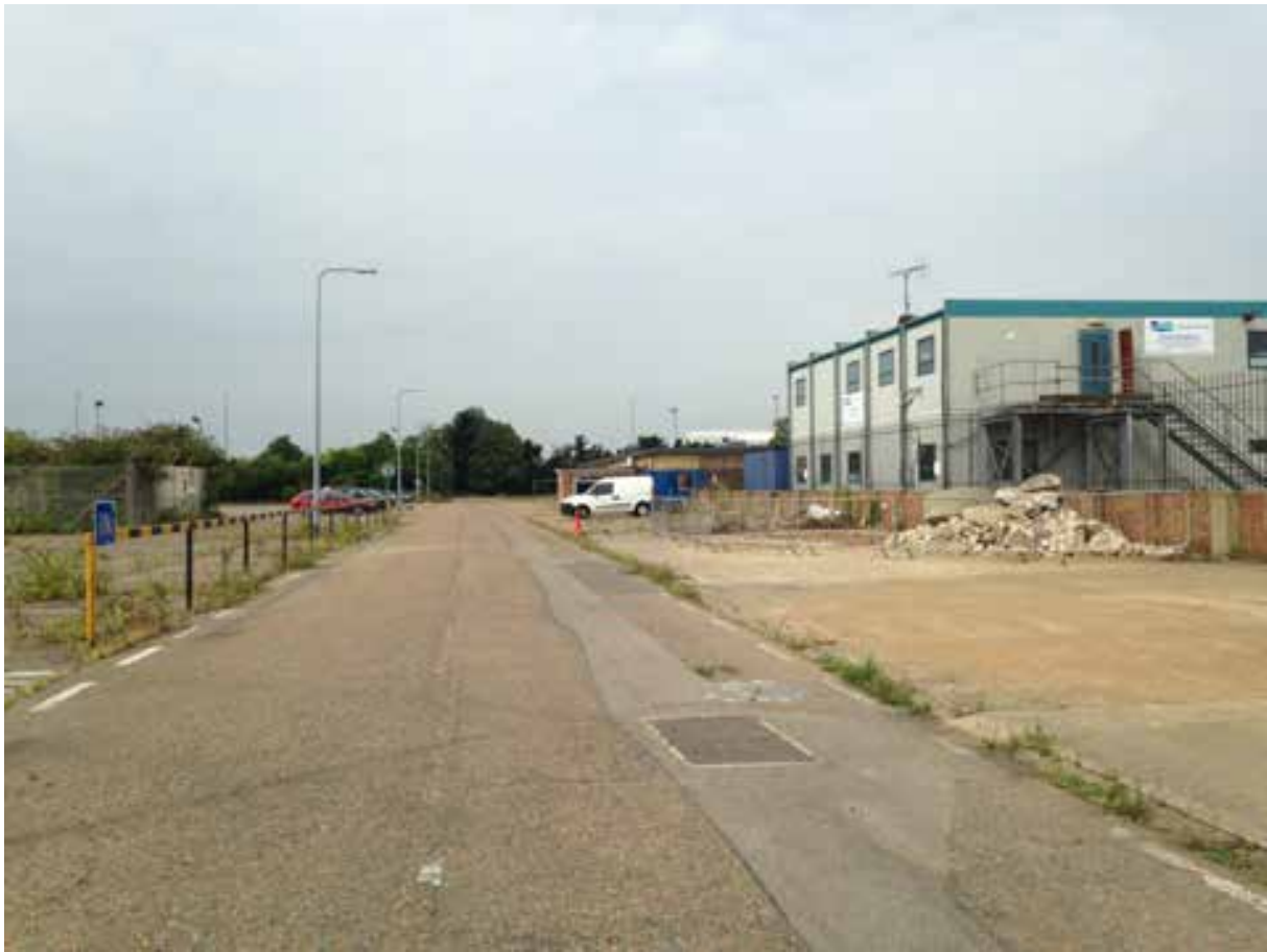
Plate 1: West facing photograph with the former Tilbury A clubhouse and temporary accommodation to the right of photograph
