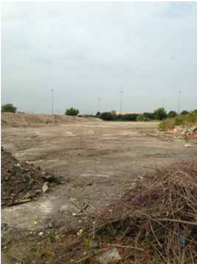
Plate 14: West facing photograph showing site clearance
