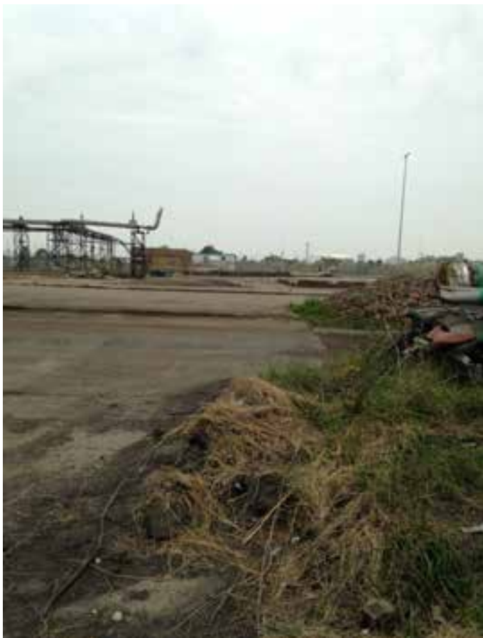
Plate 16: West facing photograph looking towards the location of the former circular tanks in the east of the site
